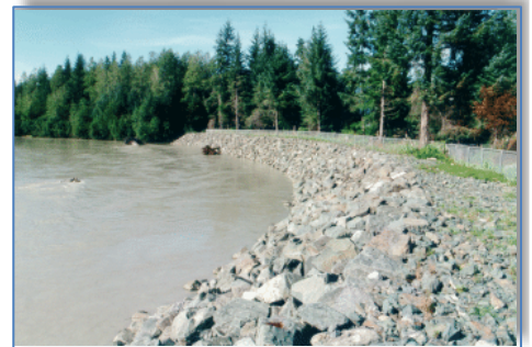
Mendenhall River Revetment Alaska
