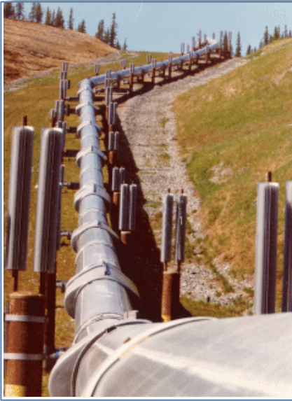
48 inch Trans-Alaska Oil Pipeline
